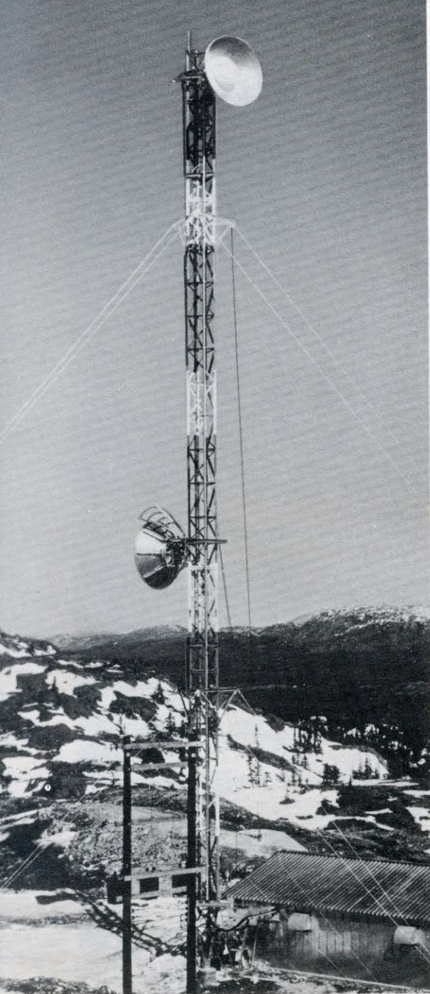
One of the stations of the Canada-Alaska microwave system built by RCA Victor Company, Ltd.
